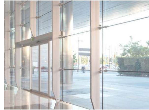
STRUCTURAL GLASS WALL W/ STRUCTURAL BACKUP
