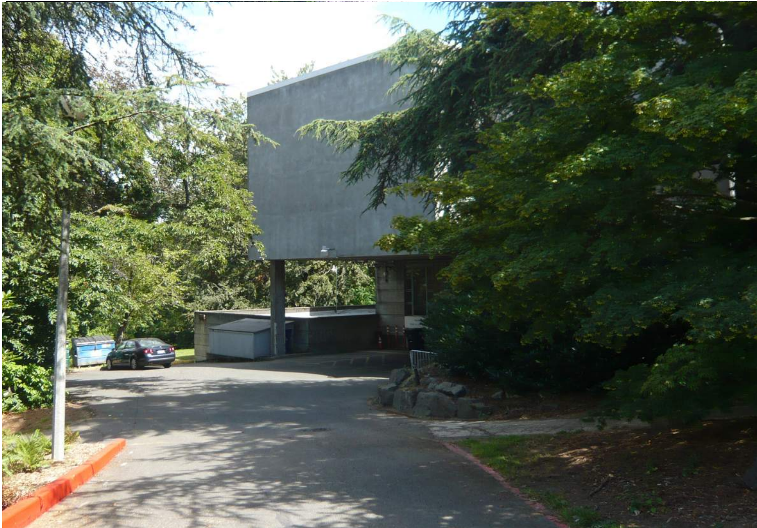
view from driveway
