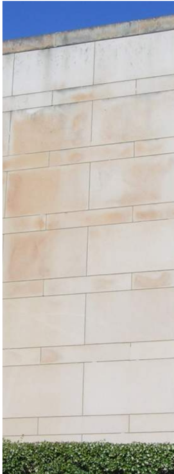
EXISTING STONE FACADE
