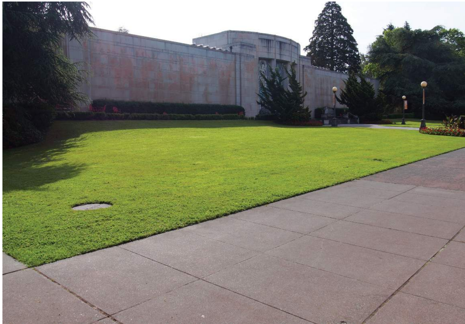
view from northwest corner
