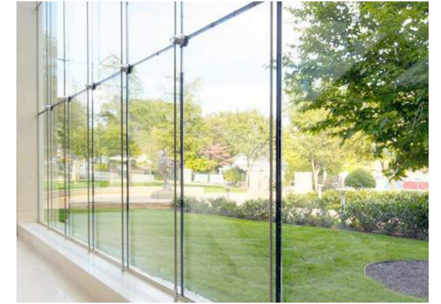
STRUCTURAL GLASS WALL
